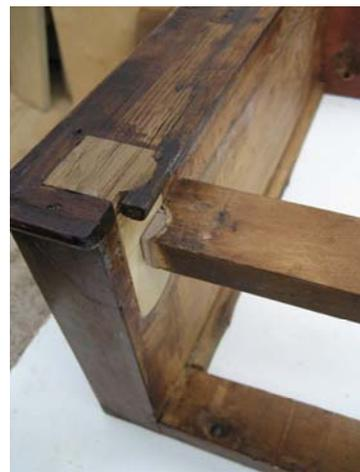
After removal of most remaining hide glue using Laponite pine (for the carcass) and oak (for the trim) was spliced into place to fill the damaged areas left by the auger drill. The splices were carved to fit the existing grooves and glued into place with hide glue.
