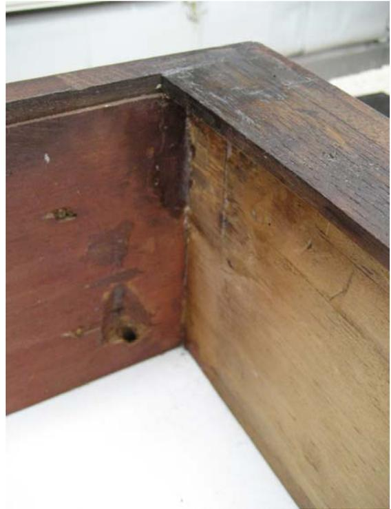
The splices were coloured in to match the existing timber using Potassium Dichromate and Oxalic acid to attain a similar base colour, then detailed using earth pigments and shellac.
